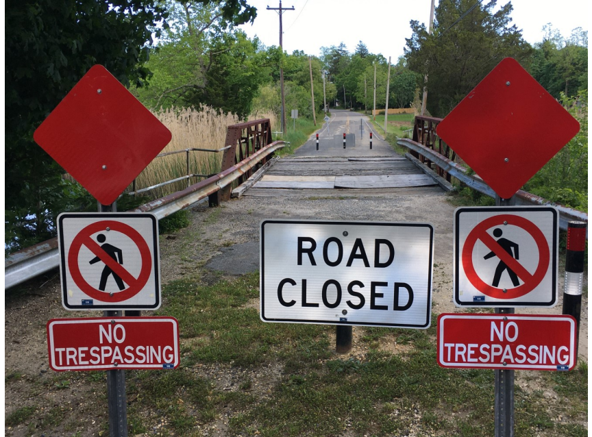
Marshallville Bridge @ Mill Creek.
